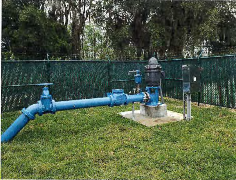
Astatula Water Treatment Plant
