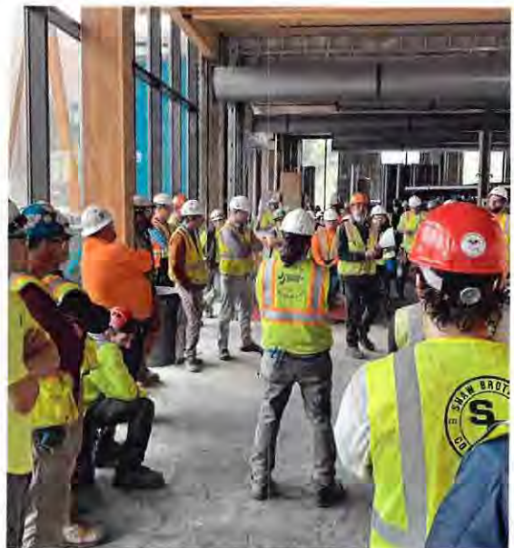
Once construction begins, PC hosts mandatory safety briefings every morning along with weekly toolbox talks.
