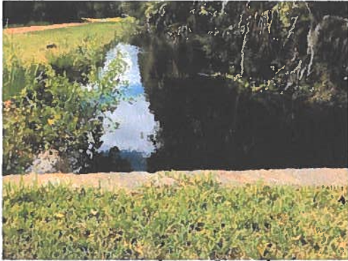
West side of culvert
