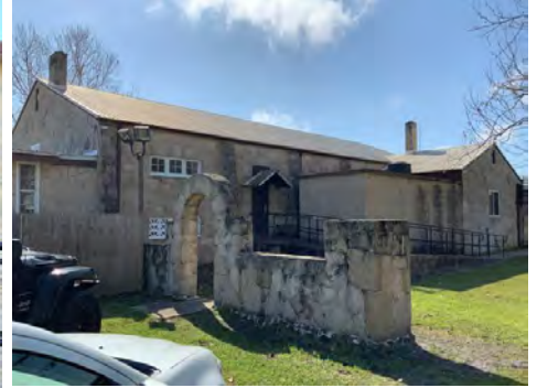
Left elevation photo number three
