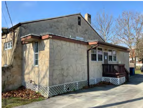
Rear elevation photo number two
