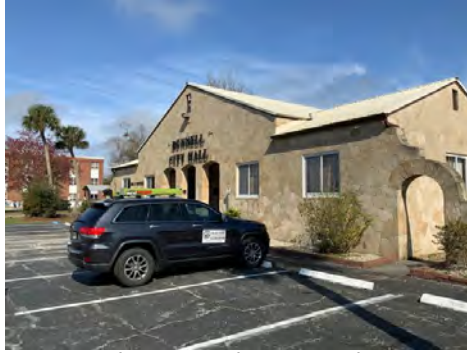
Front elevation photo number one
