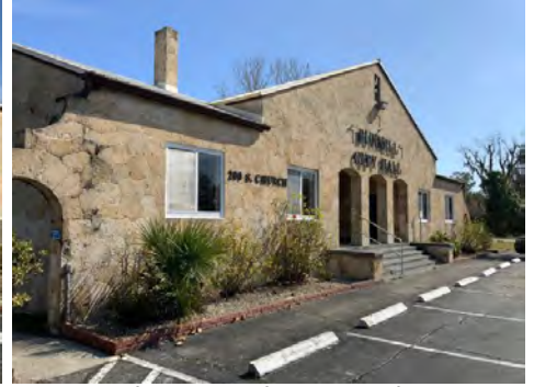
Front elevation photo number two
