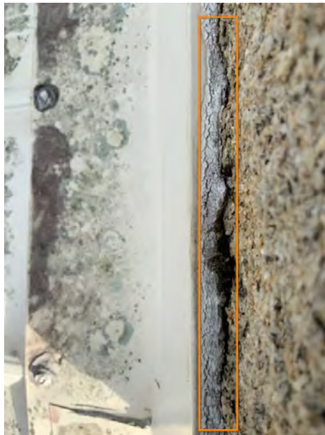
Falling sealant
