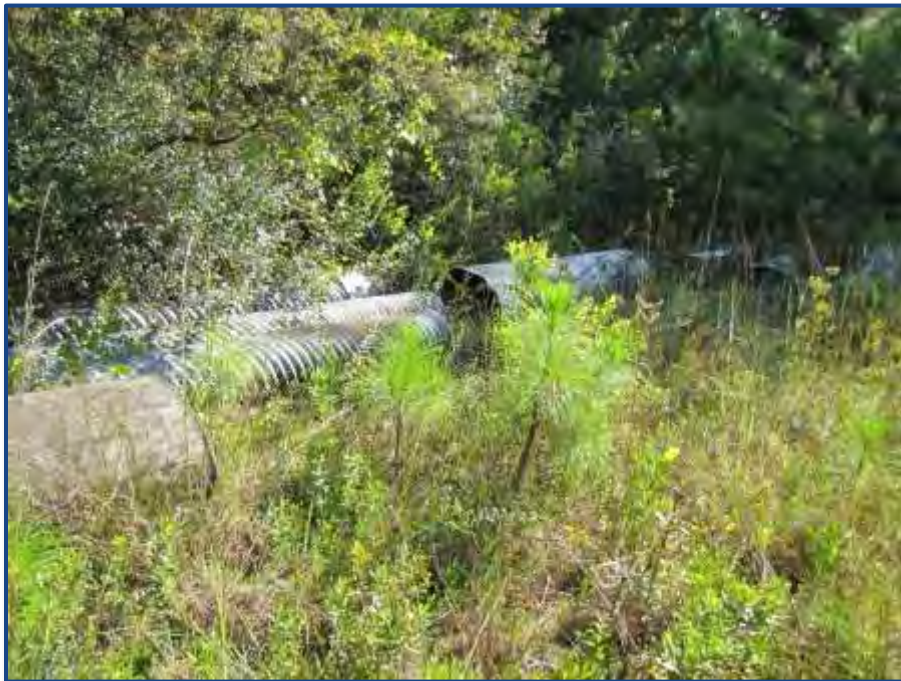
Photograph No. 14: View of drainage piping observed on the subject property
