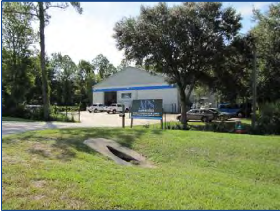
Photograph No. 17: View of Atlantic Pipe Services to the north of the subject property
