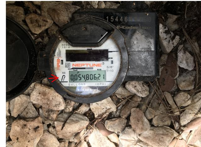
If the water faucet indicator (see red arrow) is flashing you have an intermittent leak. If the water faucet indicator is on continuously you have a continuous leak. Check for broken or damaged pipes. Sporadic leaks may not always be visible so check often.
